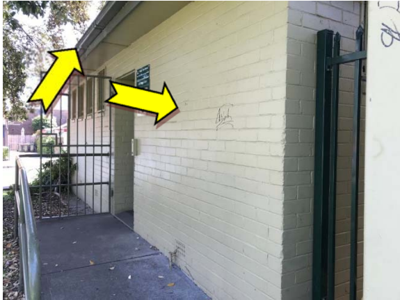
Photo 7. Exterior, throughout, walls and features – suspected lead-containing light and dark green upper coloured paint systems.
