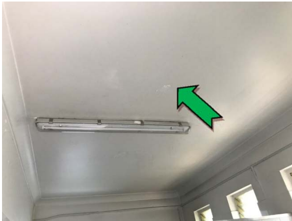
Photo 3. Interior, men's toilet, ceiling – assumed non asbestos-containing fibre cement sheeting.
