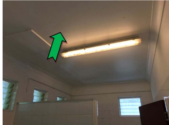
Photo 2. Interior, ladies toilet, ceiling – non asbestos-containing fibre cement sheeting.
